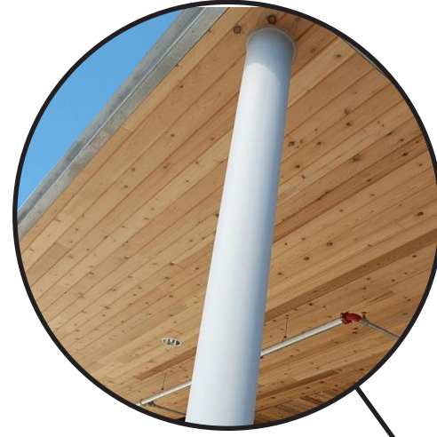
wood shiplap ceiling painted metal columns
