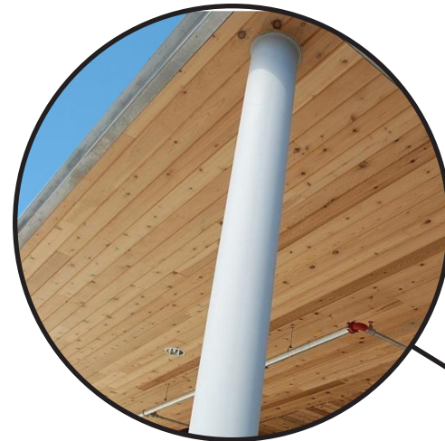
wood shiplap ceiling painted metal columns
