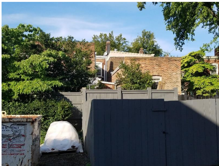
Figure 4. Rear party enclosure, view from the alley.
