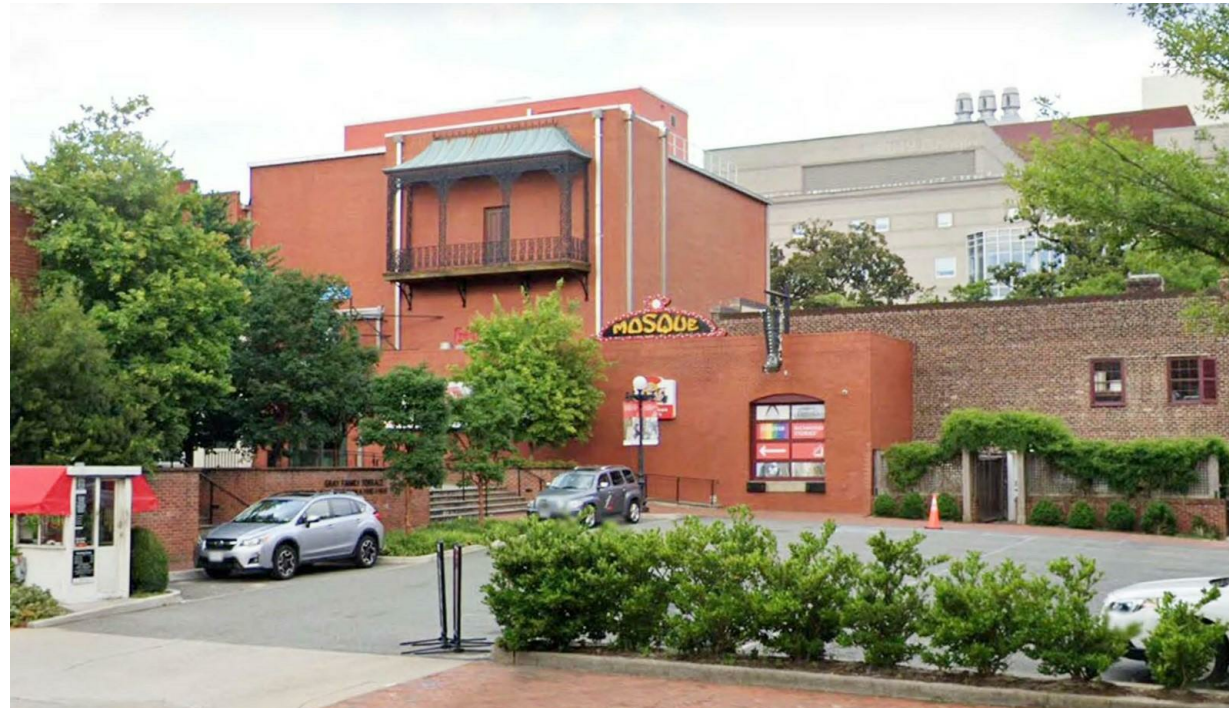
A - EXISTING - VIEW TO NORTHEAST
