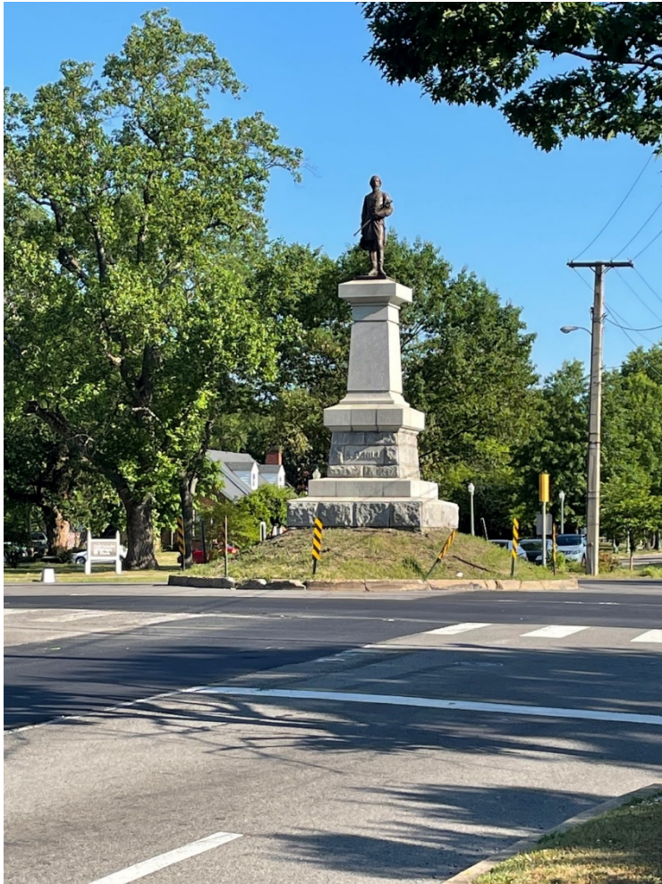
A.P. Hill Monument, current conditions
