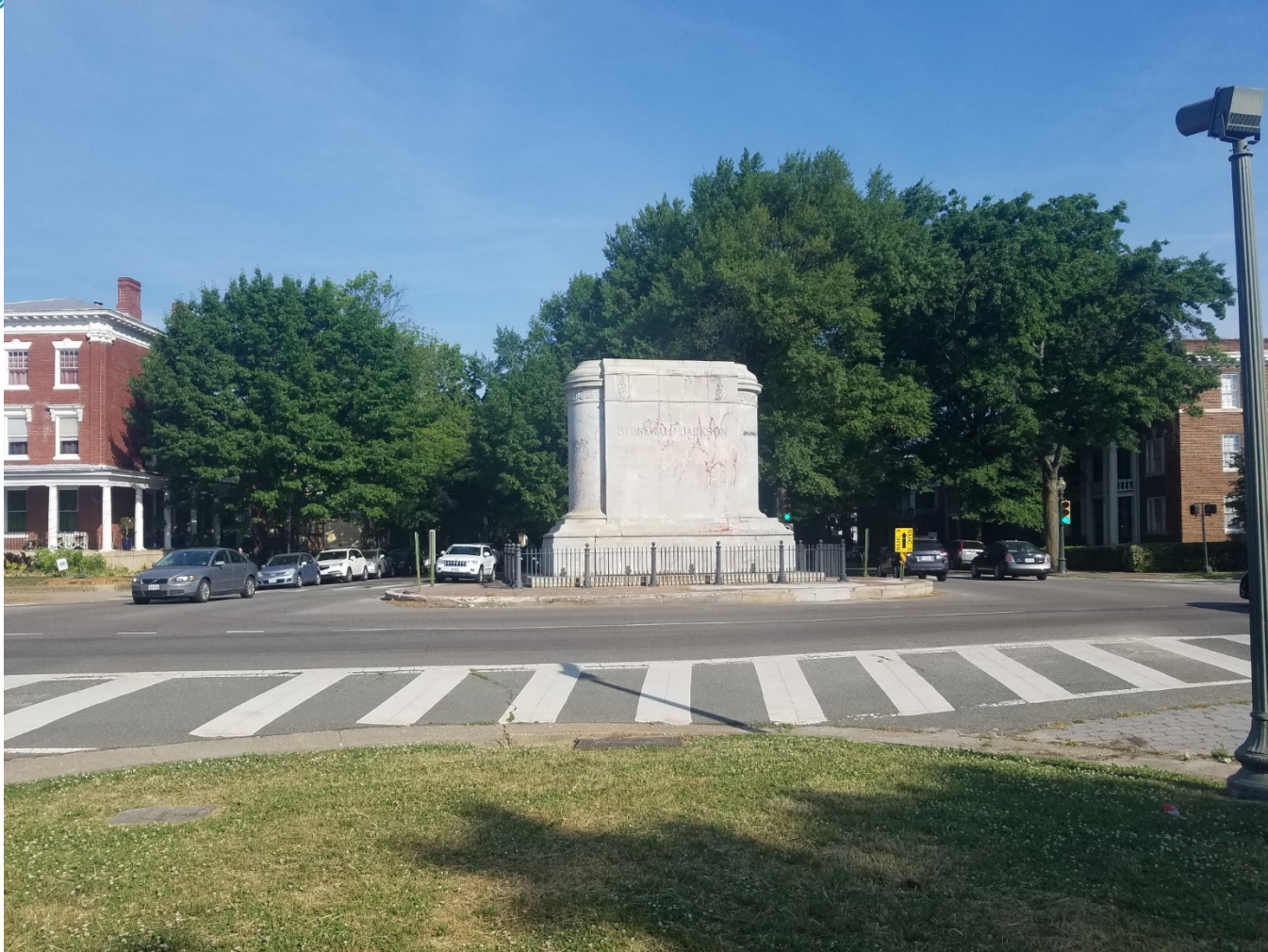
Stonewall Jackson Monument, current condition
