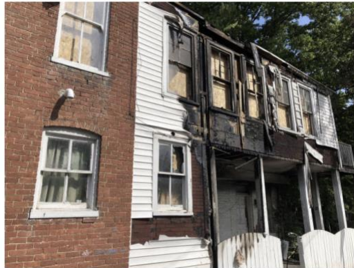
Figure 1: Fire damage at the rear of the dwelling
