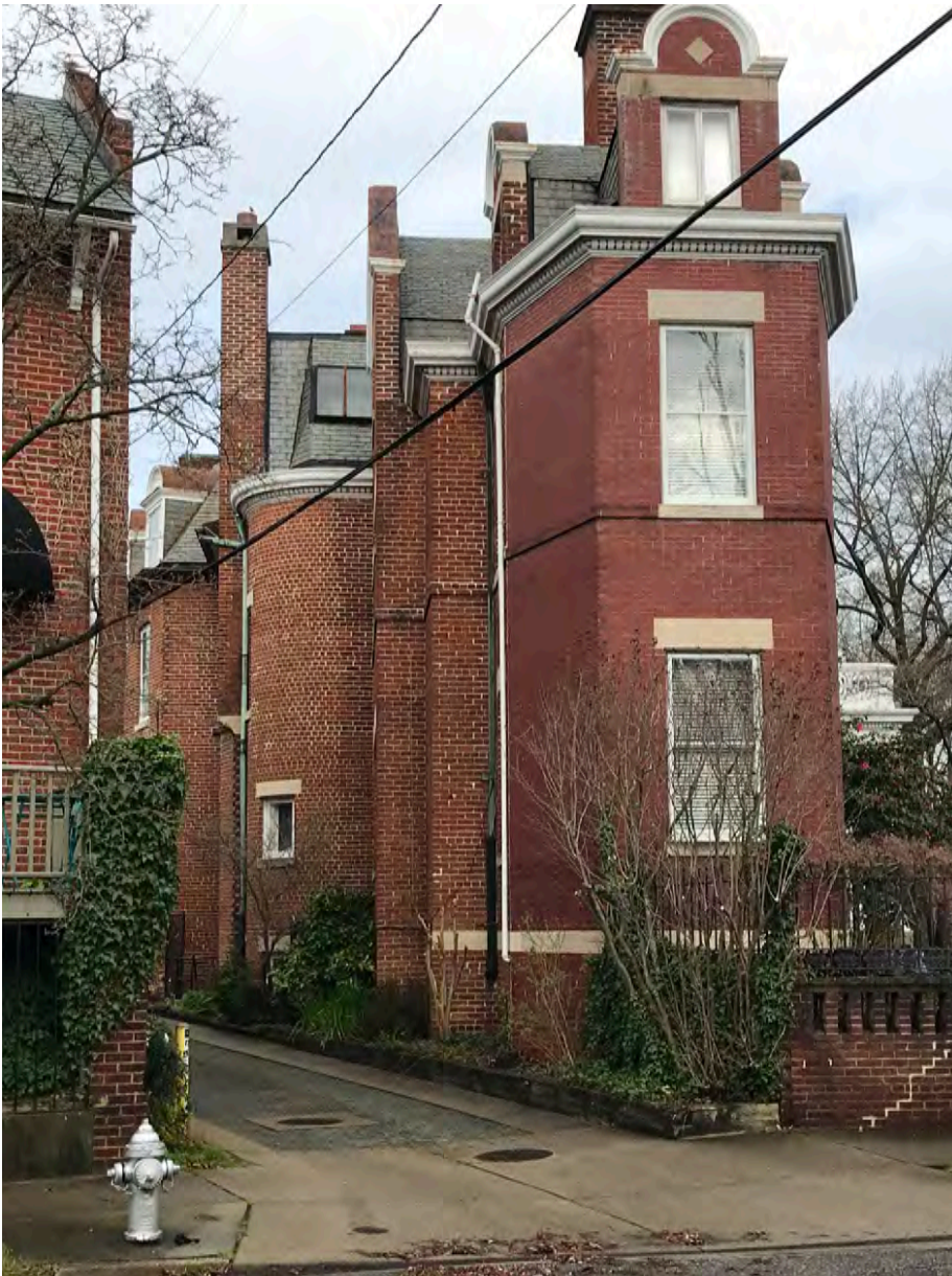
View of 3201 Monument Avenue and alleyway from Cleveland Street
