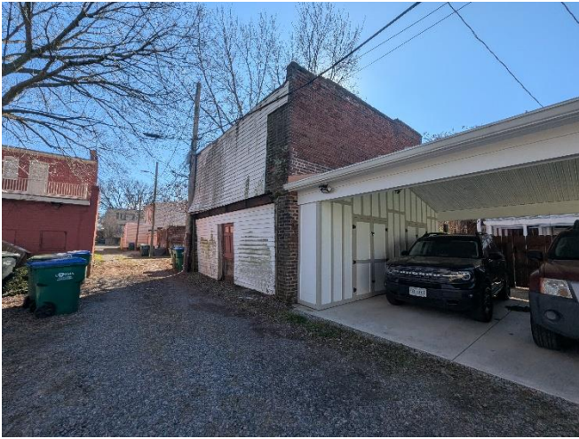
Figure 6: subject two-story carriage house
