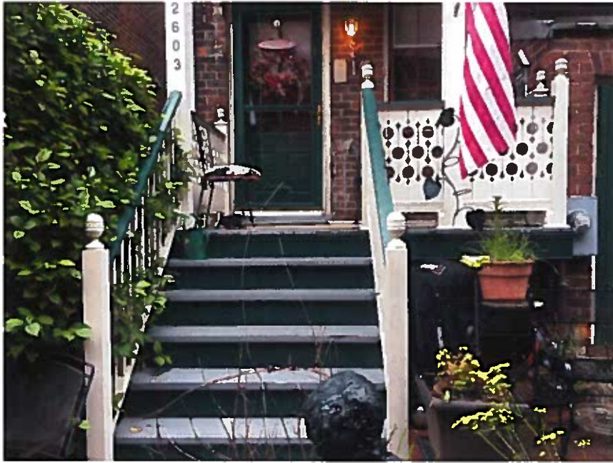
2603 East Broad Street. Upper balcony post is incorporated into landing.
