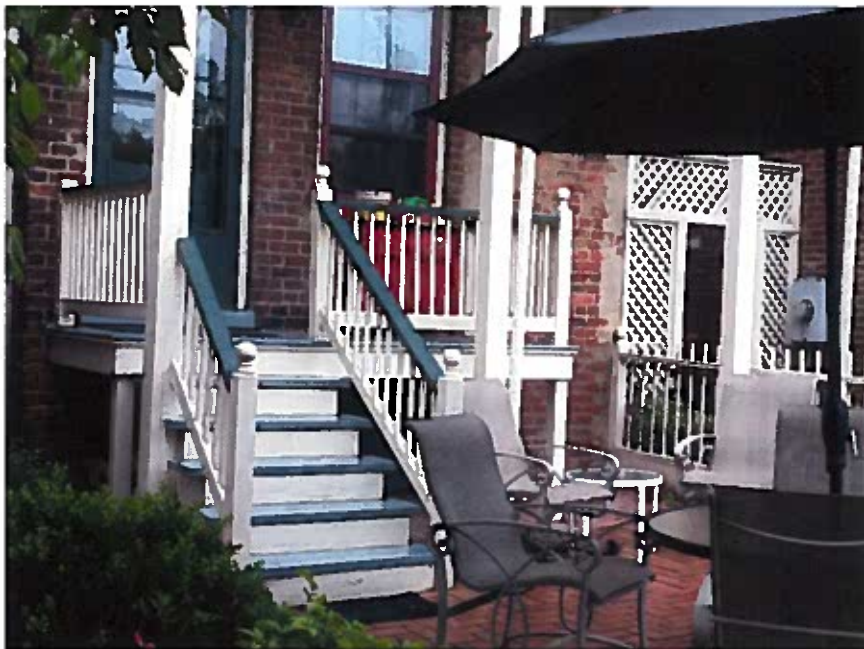
2605 E Broad Street. Upper balcony post is incorporated into the rail system.
