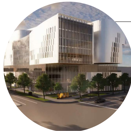
VCU Arts and Innovation Building New Construction
