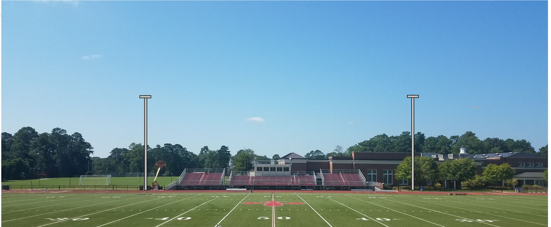
Two 80' poles located on the south side of the field
