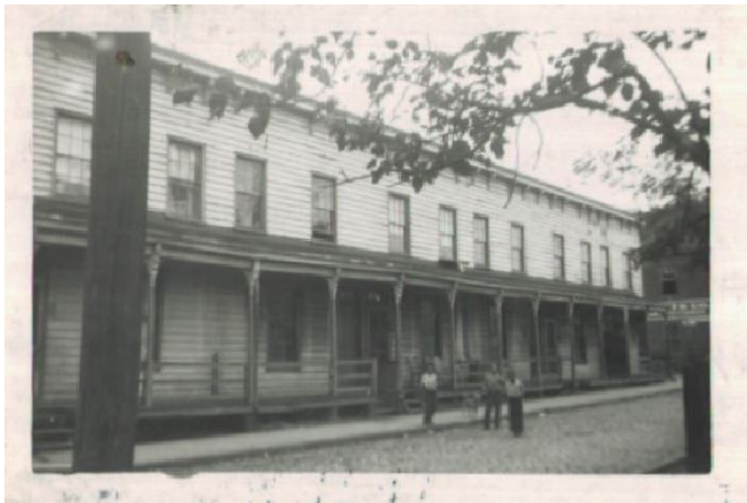
Figure 1. Assessor's Card photo showing the attached dwellings located at 2316-2326 Burton Street. The west end units are the former 2316-2318 Burton Street, the subject parcel's buildings were demolished sometime in the late 1970's or early 1980's.
