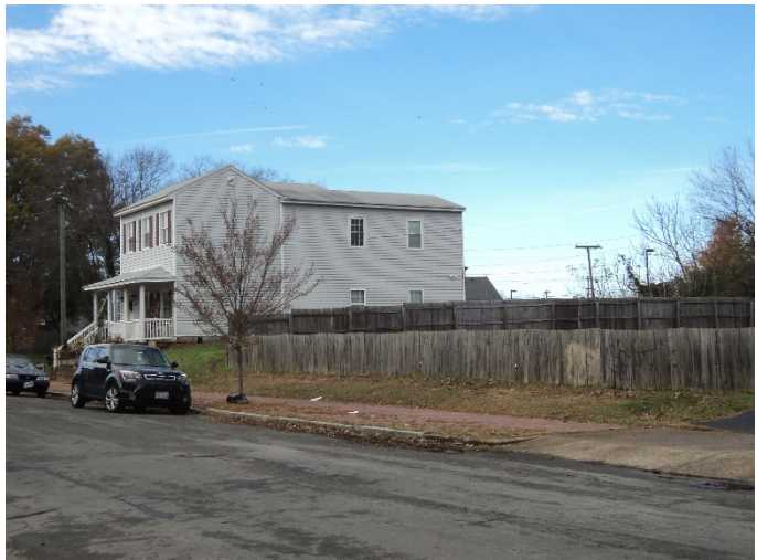
Figure 5. North side of 2200 block Cedar St., looking northwest
