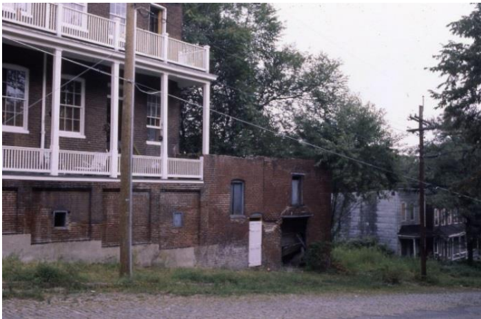
Figure 9. Former garage addition, ca. 1981.
