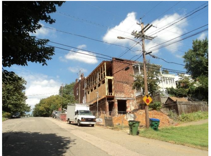
Figure 12. Side and rear elevation, August 2018.
