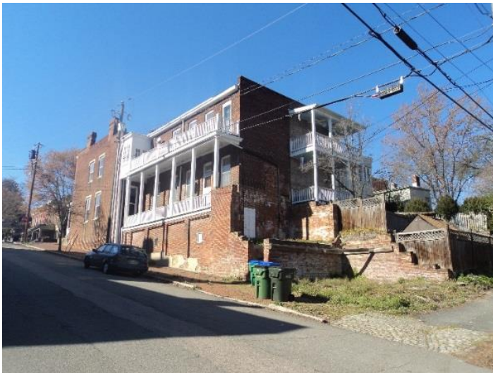
Figure 11. Side and rear elevation, March 2017.
