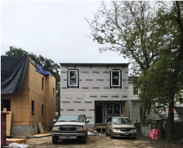
Figure 1. 2113 Cedar Street, rear.
