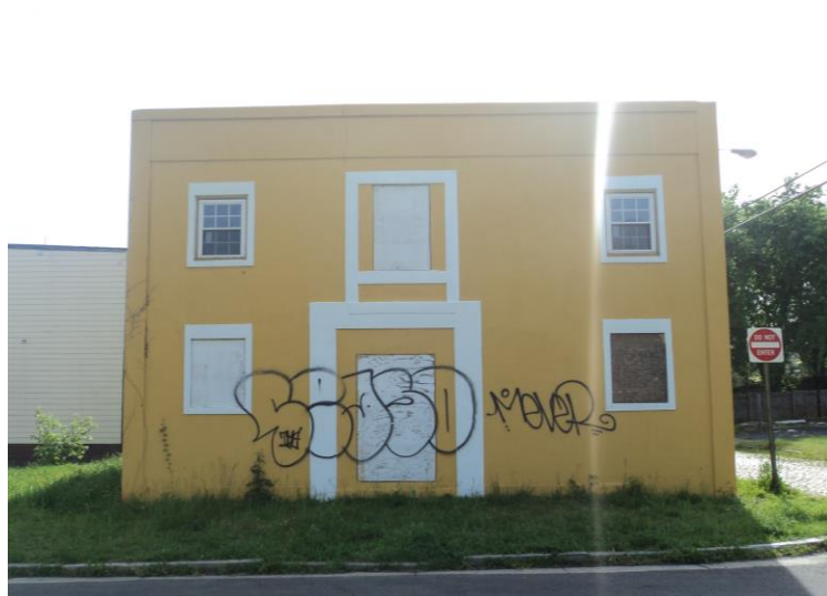
Existing Condition of the Façade of 815 North 22 nd Street
