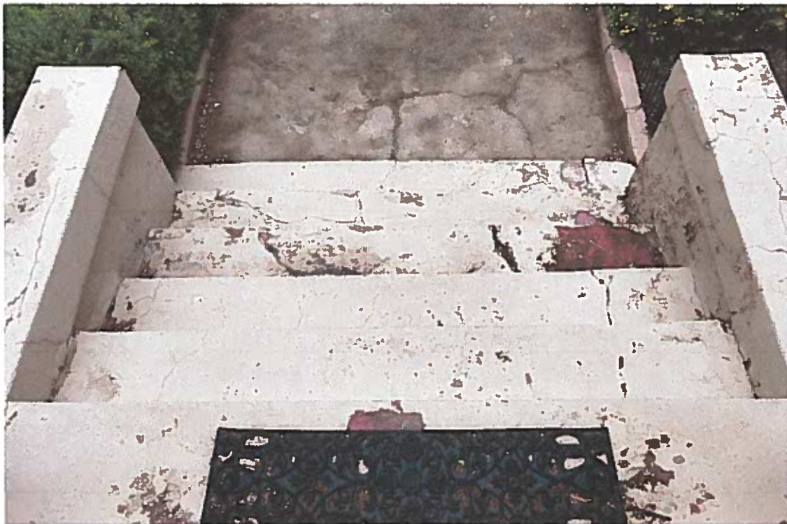
Front Stairs Viewed Downward From Porch
