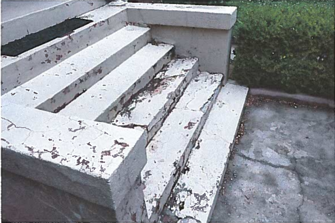
Front Stairs Viewed From Side
