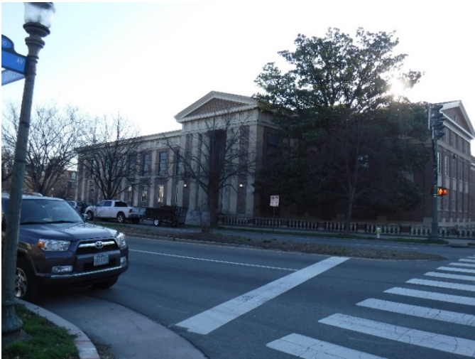
Figure 3. First Baptist Church, looking east
