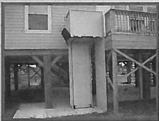
Porch Landing - Elevated Residence with Platform Gate
