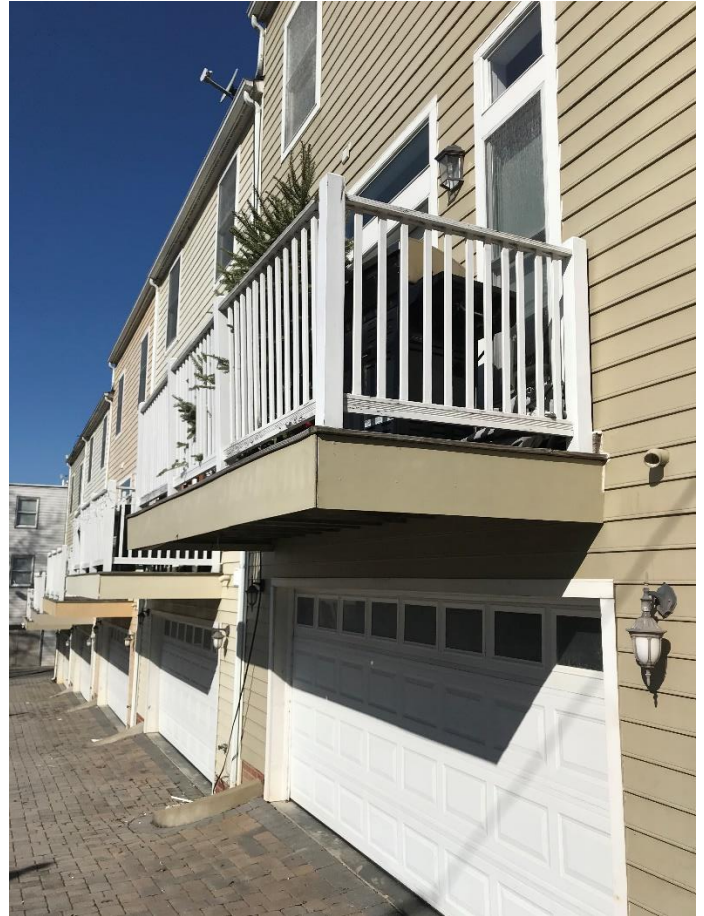
Figure 2. Rear deck detail
