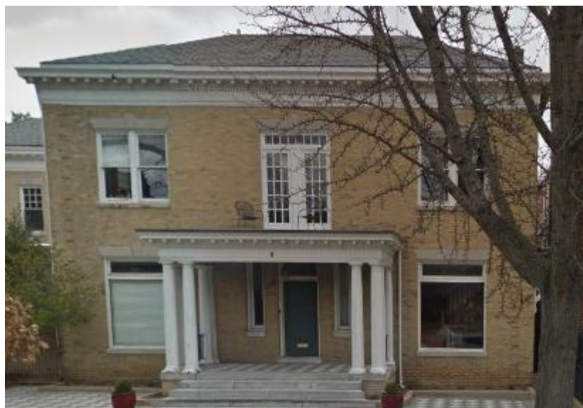
1208 W. Franklin Street, February 2016 (Source: Google street view)
