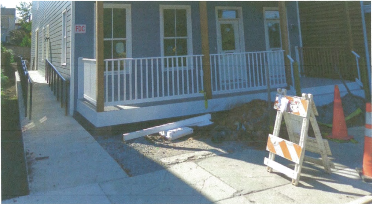
Example of a similar ramp at a recent project
