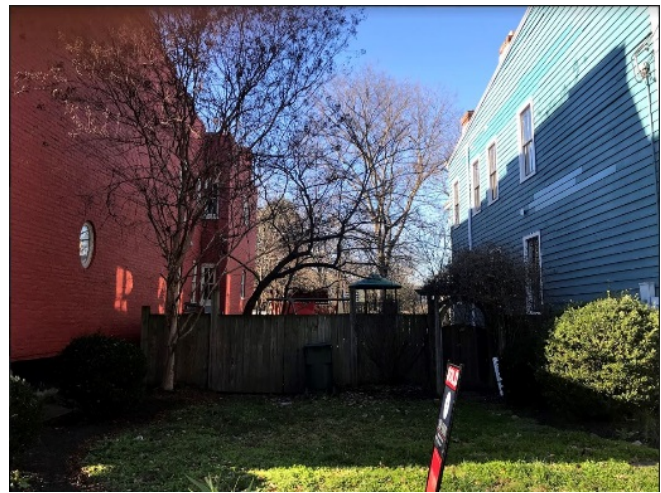
Figure 4. 312 North 32nd Street, current conditions.
