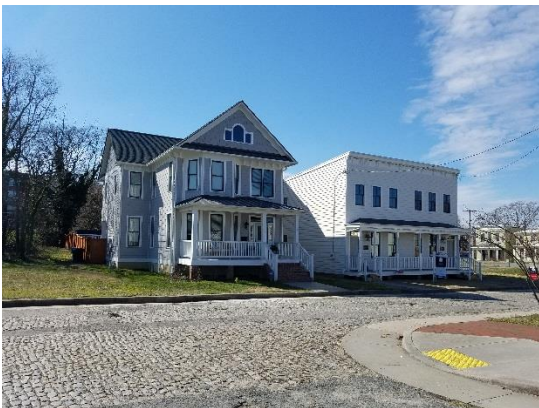
Figure 5. 2313-2315 and 2317 Carrington Street.
