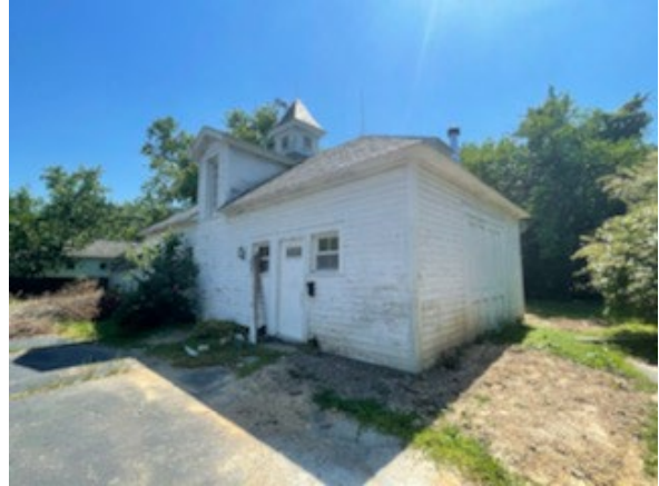
Figure 2. 4002 Existing Rear Carriage House, 2021. Hipped roof with through-the-eave dormer and cupola. (pre-rehabilitation).
