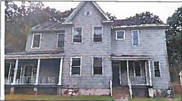
Side elevation – note concrete steps to porch
