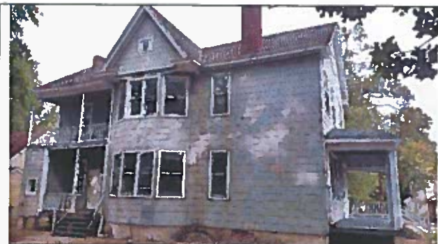
Rear elevation – note wooden side steps
