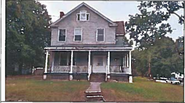
Front elevation – note concrete steps to porch
