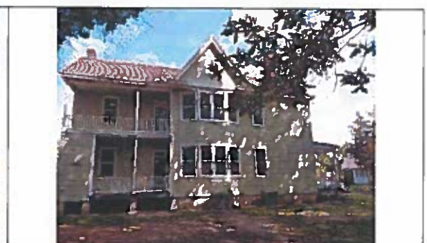
Rear elevation – note side steps removed
