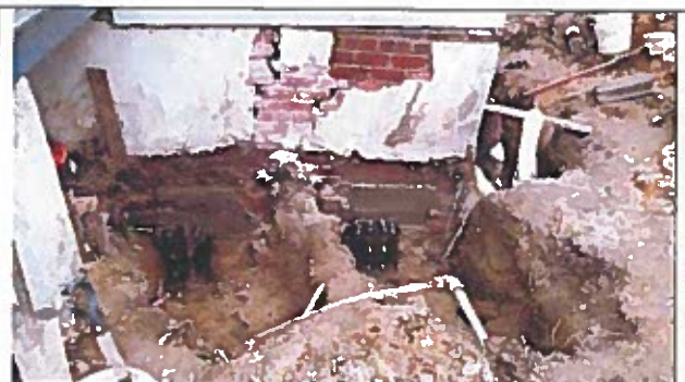
Foundation repair – east side (note two helical piers)
