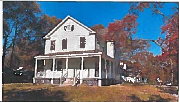
Front elevation – concrete spalling repaired
