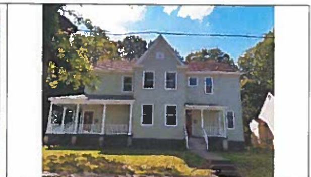
Side elevation – concrete spalling repaired
