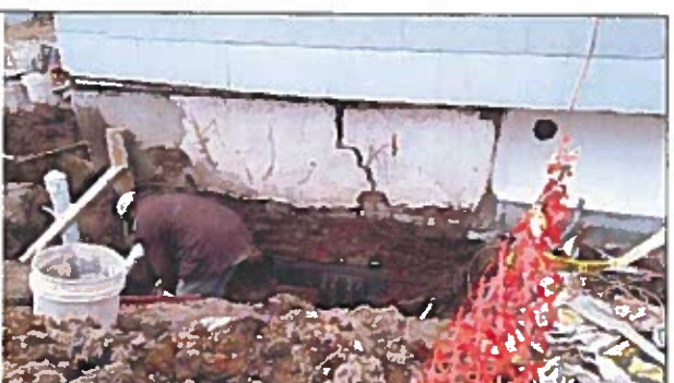
Foundation repair – north side (note two more helical piers)
