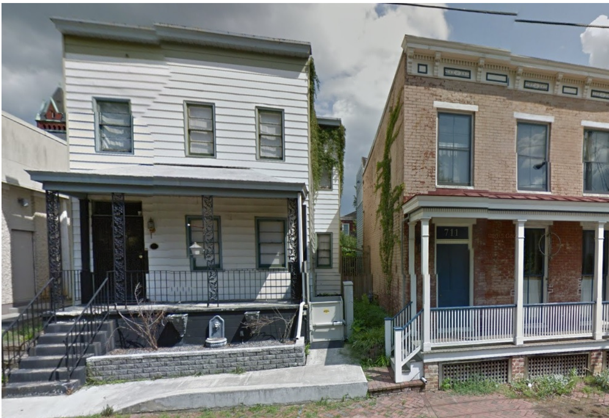
700 Block of 23 rd st. Recessed bay on the right.
