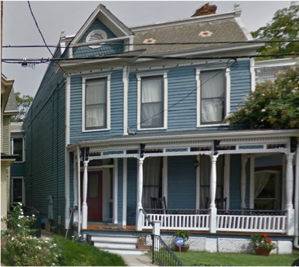
3600 Block of E. Broad. Recessed additional bay on the left.
