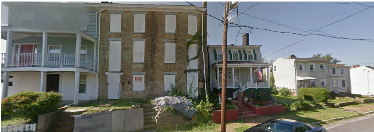
2100 Block of Cedar St. Mix of 2 story houses and 3 story houses.
