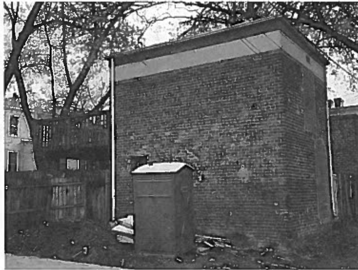
3310 E Broad Street: Two-story carriage house
