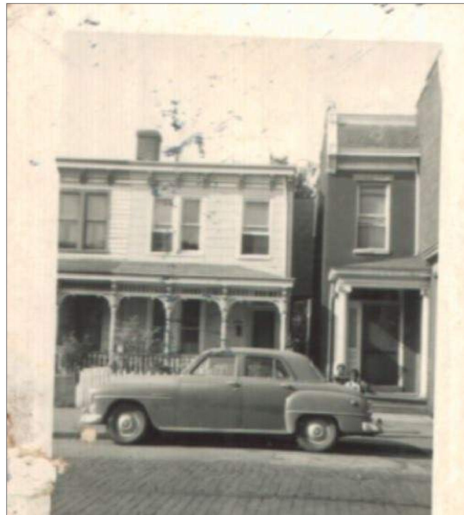
Historic Front Elevation of 3103-3105 East Marshall St.
