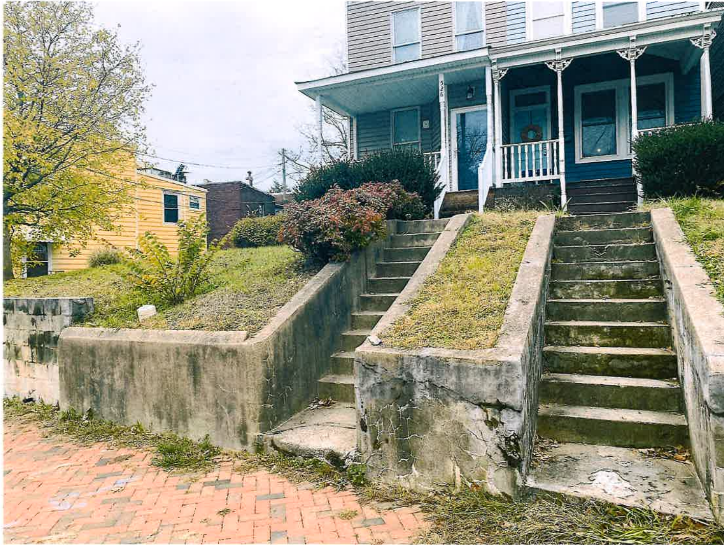
Steps leading to 526 and 528 N 21 st St. Similar steps to be cut into the retaining wall at 524 N St w/ brushed concrete path leading to the door.
