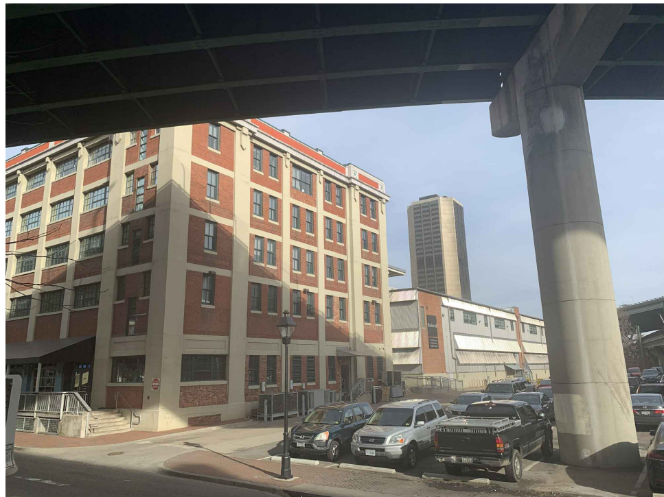
3 Existing Building - Dock Street and Drive Aisle
