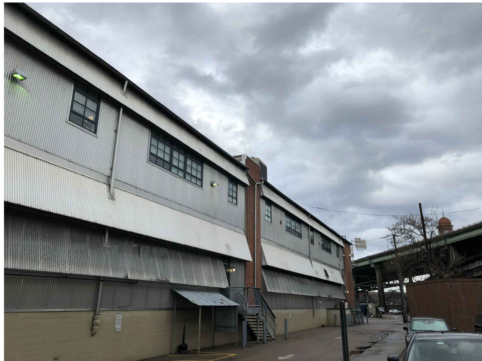
1 Existing Building - Drive Aisle
