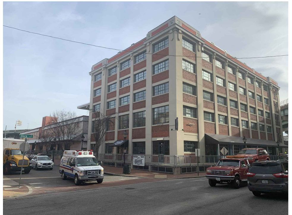
4 Existing Building - Dock Street and 15th Avenue
