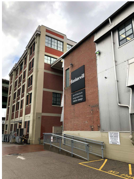
2 Existing Building - Drive Aisle
