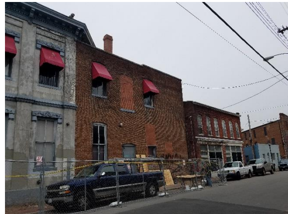
Figure 4. 200 West Marshall Street, rear section on Brook Road.
