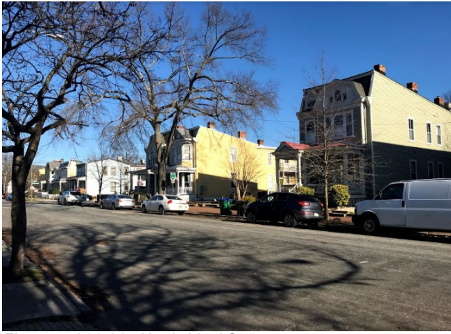
Figure 7. 311-317 North 32nd Street.
