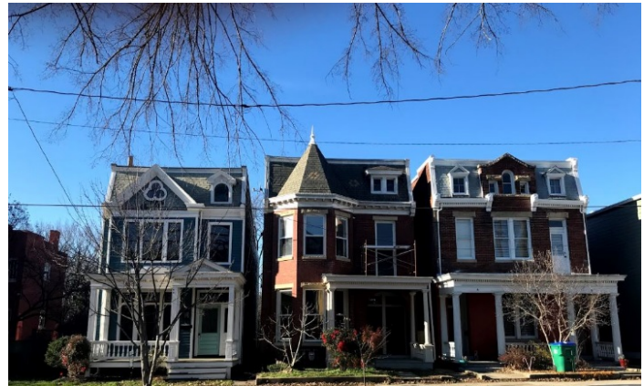
Figure 6. 314-318 North 32nd Street.
