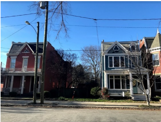
Figure 5. 310-314 North 32nd Street.
