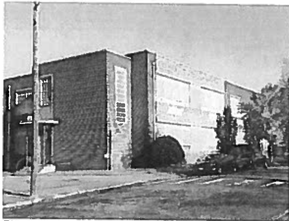
Figure 5. Existing Building, Addition.
