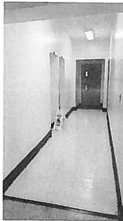
Figure 11. Non-ADA compliant bathroom corridors and spaces, ca. 1922 section
