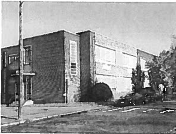
Figure 5. Existing Building, Addition.
