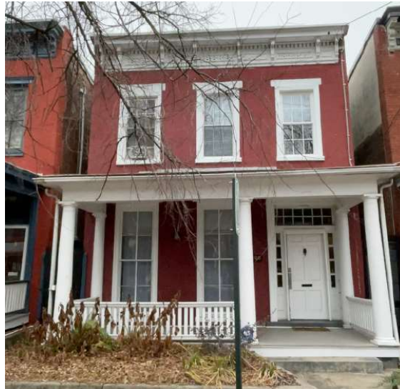
Figure 2. Current façade photo.
