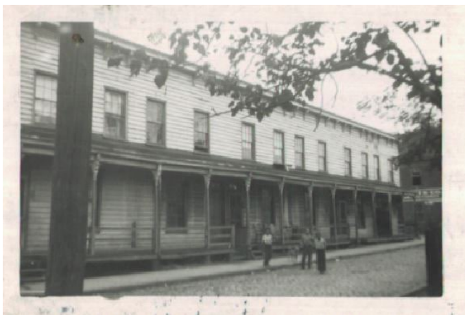
Figure 1. Assessor's Card photo showing the attached dwellings located at 2316-2326 Burton Street. The west end units are the former at 2316-2318 Burton Street, the subject parcel's buildings were demolished sometime in the late 1970's or early 1980's.
