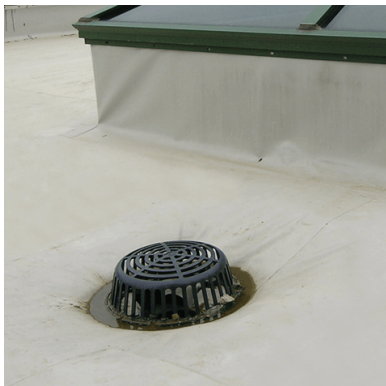
Internal Concealed Drainage System
