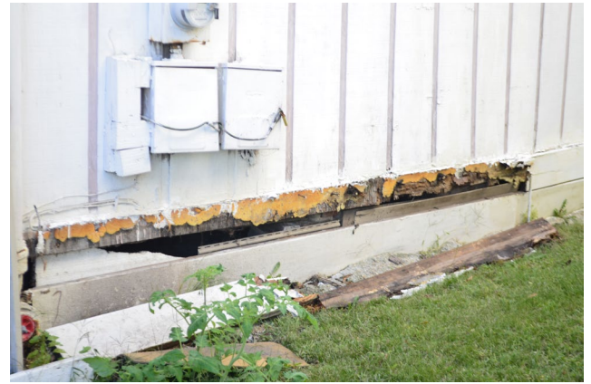
Figure 6. View of the poor condition of the foundation on the west side of 2417 Carrington Street.
