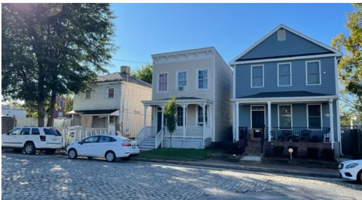
Figure 3. View of 2417, 2415 and 2413 Carrington Street.
