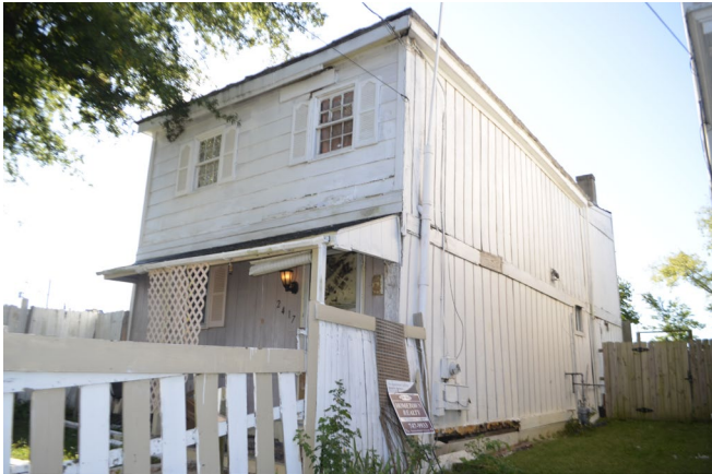
Figure 1. Existing Dwelling at 2417 Carrington Street
