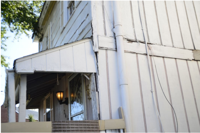
Figure 7. View of the poor condition of the siding and porch roof on the west side of 2417 Carrington Street.
