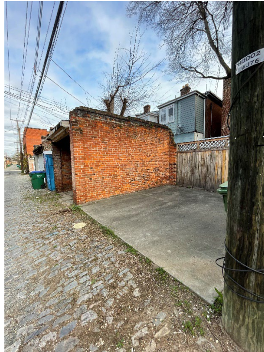
Figure 4. View of the neighboring garage at 1845 West Grace Street, which will abut against the west side of the new ADU.
