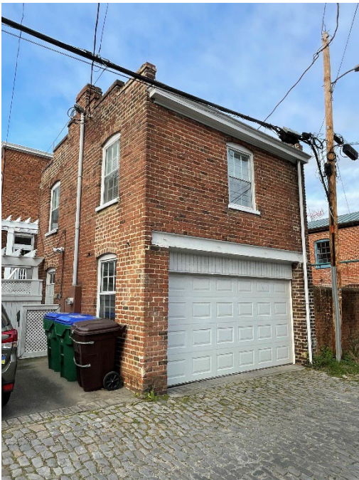
Figure 5. Garage located on the south side of the alley, for 1832 Monument Avenue. This is an example of a two-story brick garage in the vicinity, with vertically aligned windows.
