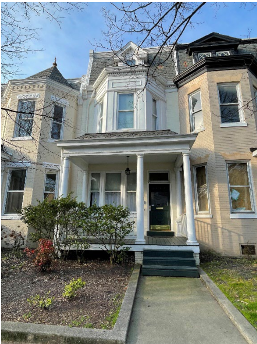
Figure 1. Photograph of the façade of 1843 West Grace Street
