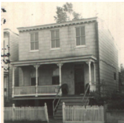
Figure 1. 2211 Venable Street, 1950s. City Assessor. Original porch posts, railings, and two over two windows in place.
