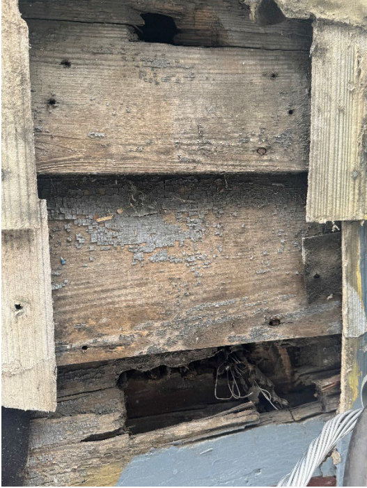
Figure 5. Original siding under aluminum siding. Poor condition with some rot and many nail punctures.
