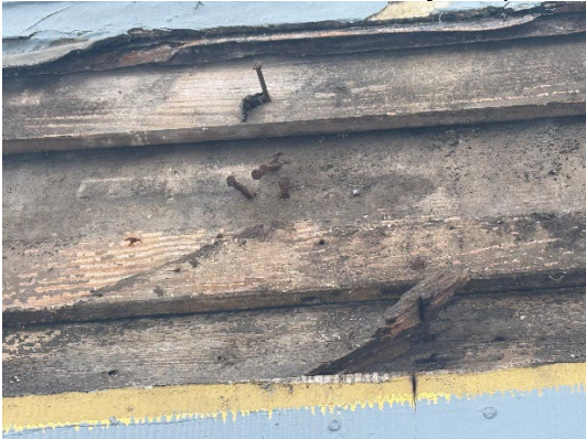
Figure 5. Original siding under aluminum siding. Poor condition with some rot and many nail punctures.
