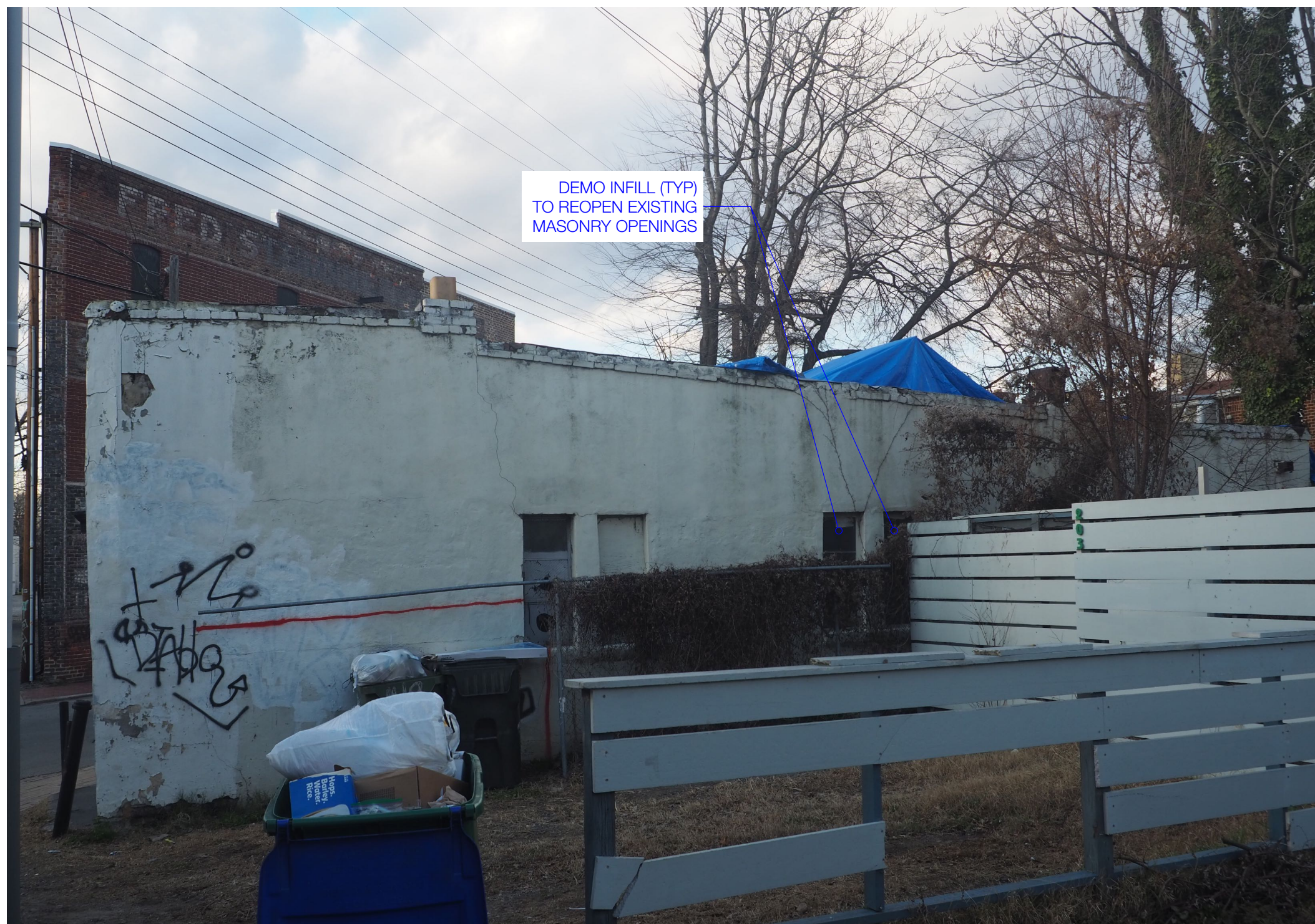
2 EXISTING / DEMO ALLEY ELEVATION SCALE: 1/4" = 1'-0" 0 2 4 6
