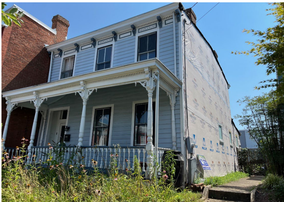
Figure 1. Existing Conditions -Façade with wood siding, sides and rear being replaced with Hardiplank.
