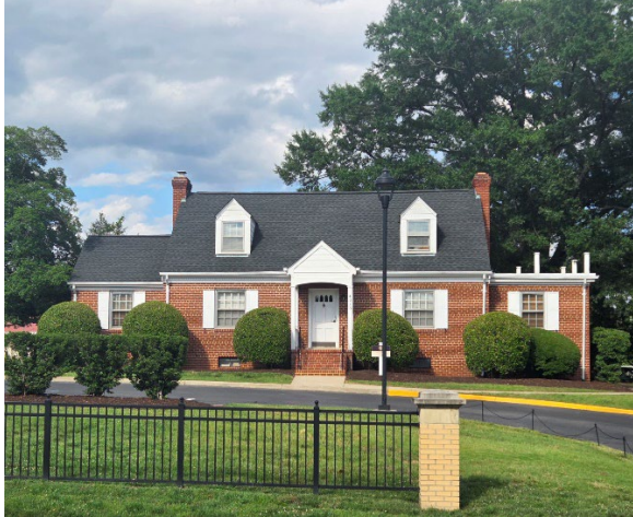
Fig. 2 – View from West
