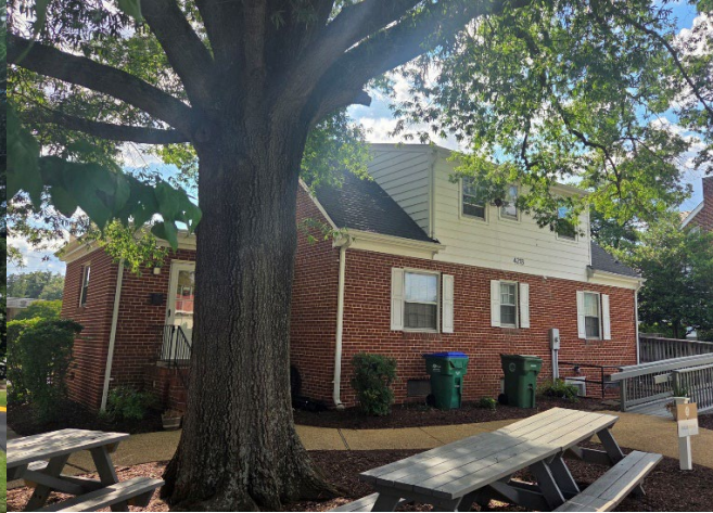
Fig. 3 – View from East
