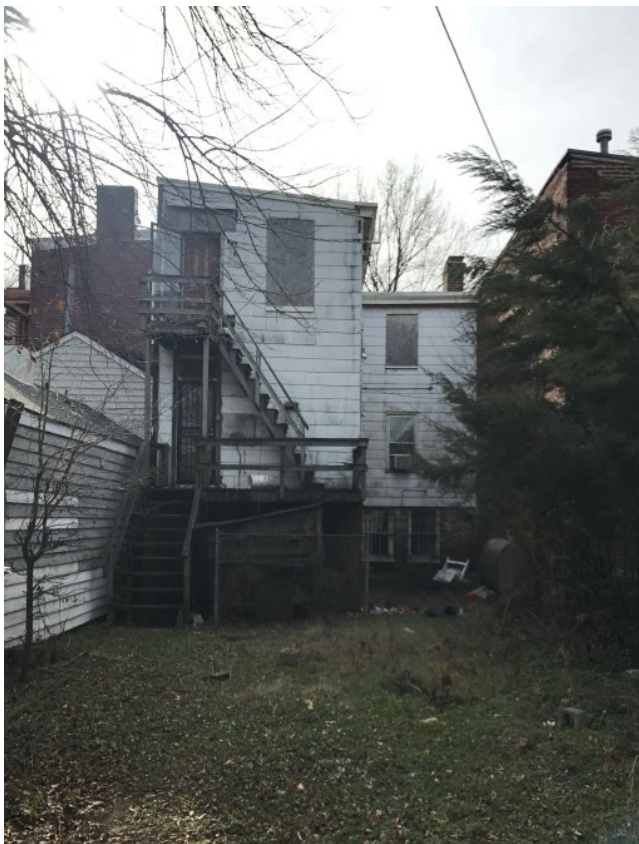
Figure 9. Rear view of 514 West Marshall Street, March 1, 2019.
