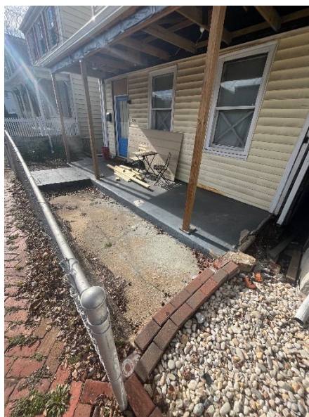
Figure 2. Front porch concrete slab and slender wooden posts.
