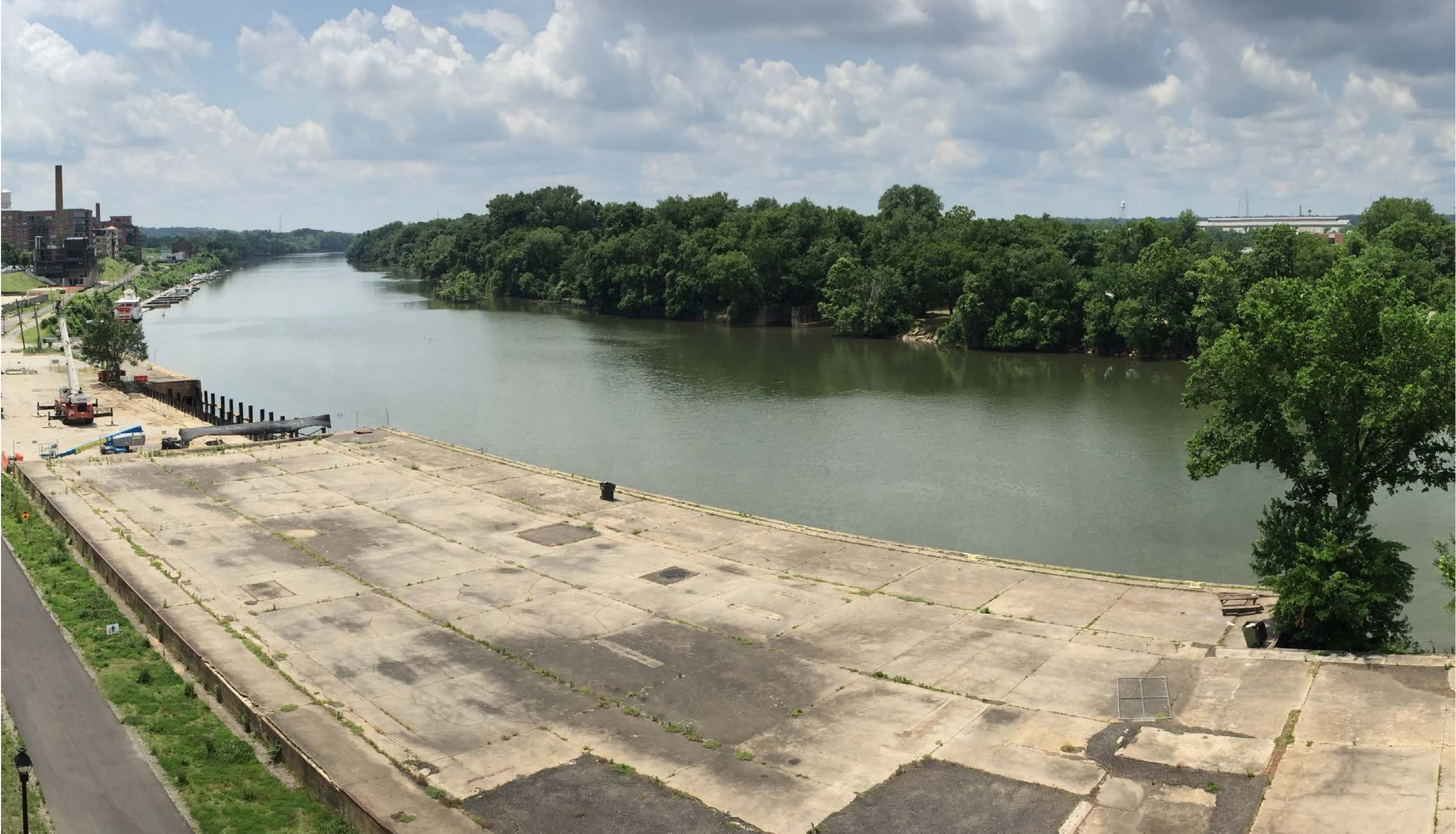
DOWNRIVER EXISTING CONDITIONS
