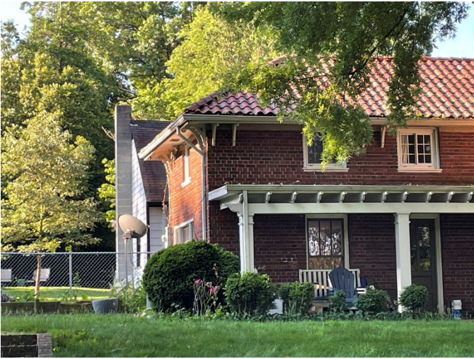
Figure 5. View of the garage's north and east elevations from Princeton Road.
