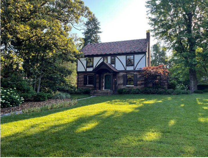
Figure 1. View of the façade of 4107 Hermitage Road.
