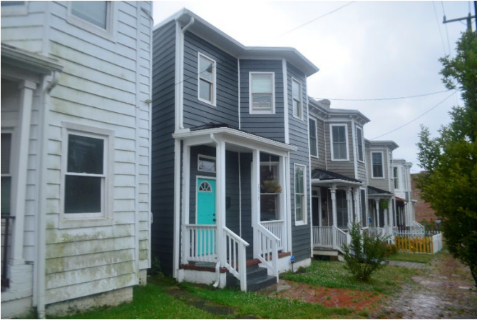
Figure 1. View of 2017 Venable Street. This house was built in 1888.
