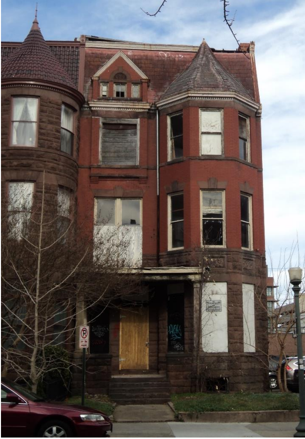
Figure 1. 2006 W Franklin St, facade
