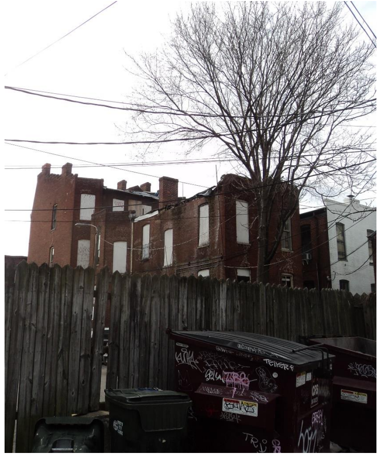
Figure 2. Current view of rear and side elevation
