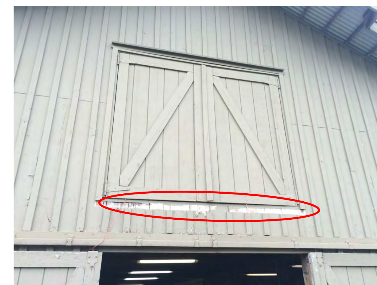
3. REPLACE SILL AT NORTH BARN LOFT DOOR
