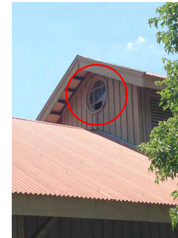
8. REPLACE BROKEN PANE AT EXISTING BATHROOM EAST ROUND MONITOR WINDOW
