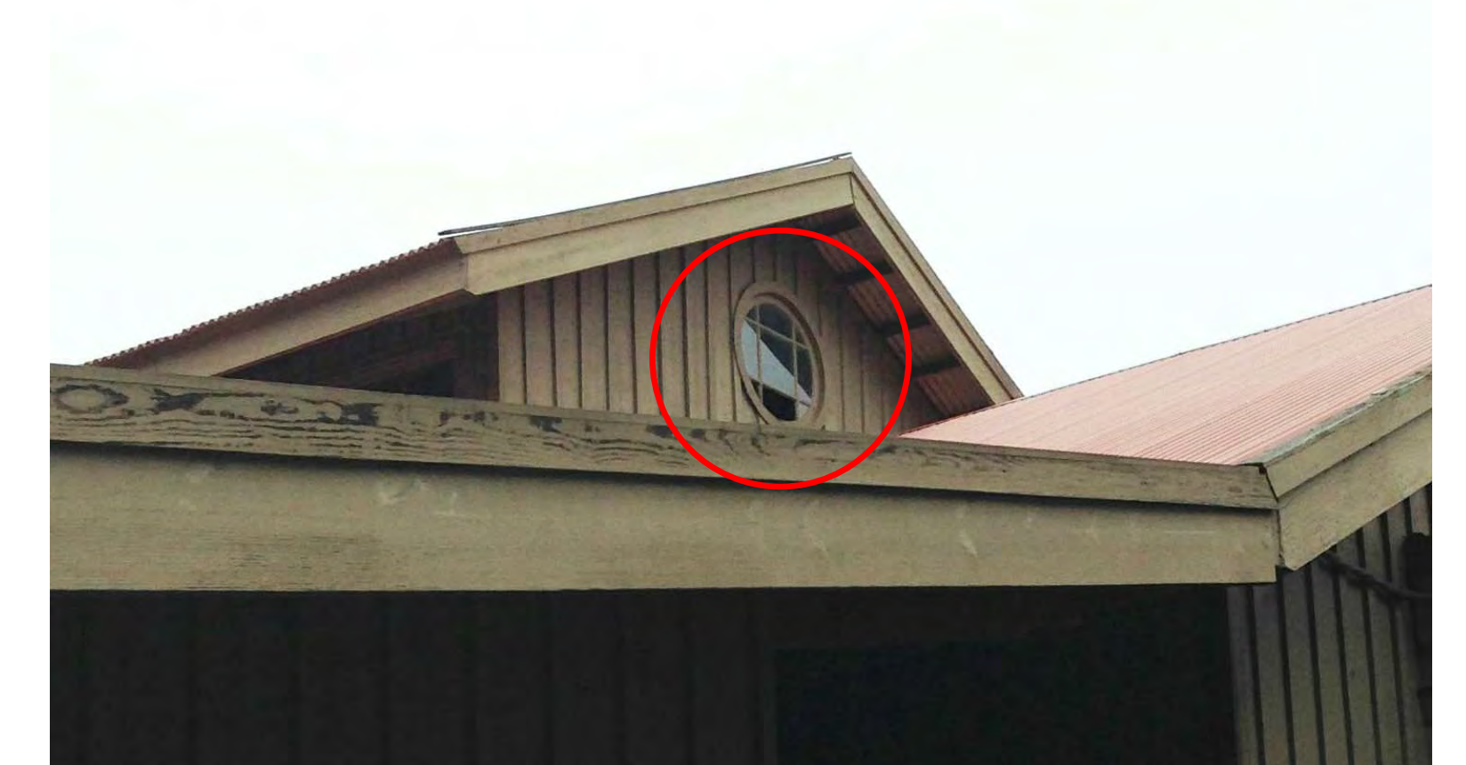
7. REPLACE BROKEN PANE AT EXISTING BARN SOUTH ROUND MONITOR WINDOW
