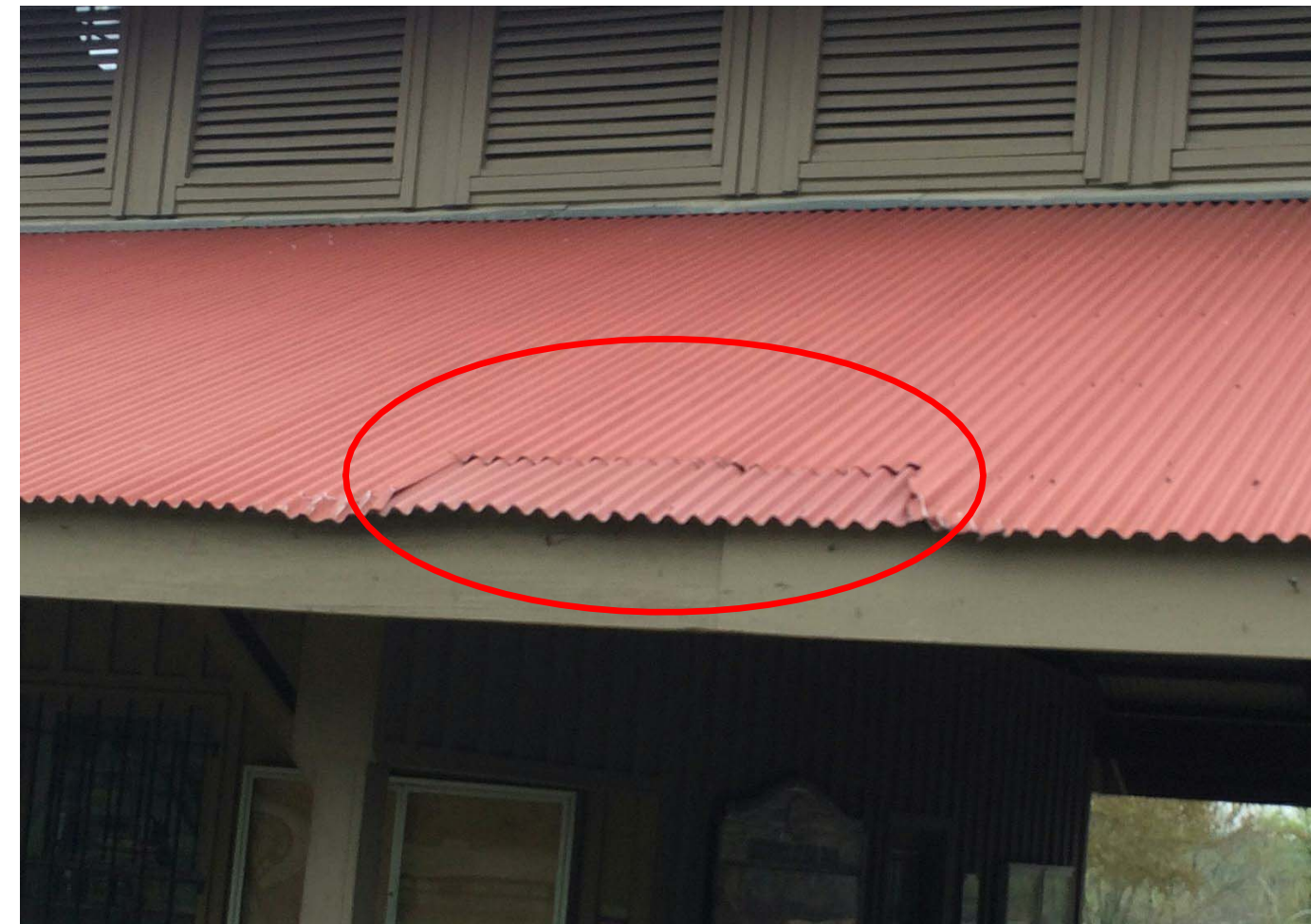
11. REPAIR ROOF AT PATCH NEAR EXISTING BATHROOMS
