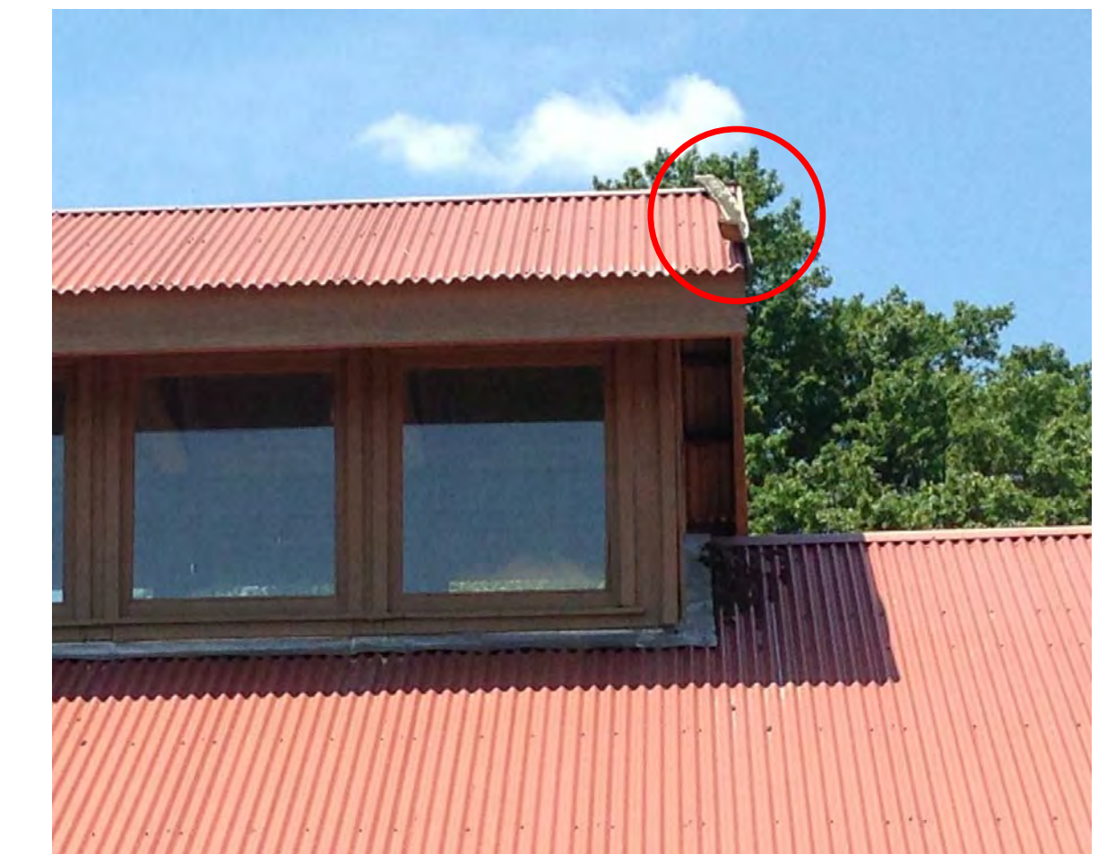
6. REPAIR ROOF AT NORTH GABLE END OF EXISTING CLASSROOM MONITOR
