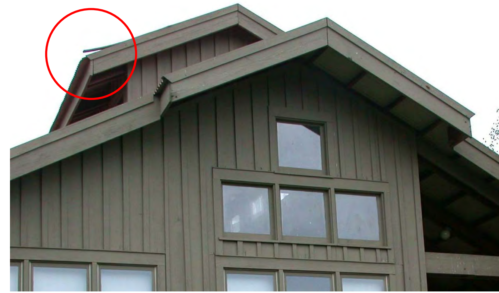
10. REPAIR ROOF AT SOUTH GABLE END OF EXISTING CLASSROOM MONITOR
