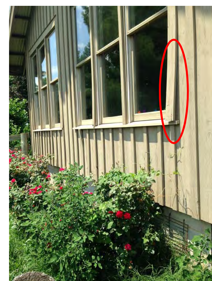
5. REPLACE CASING AT EXISTING CLASSROOM SOUTH WINDOWS
