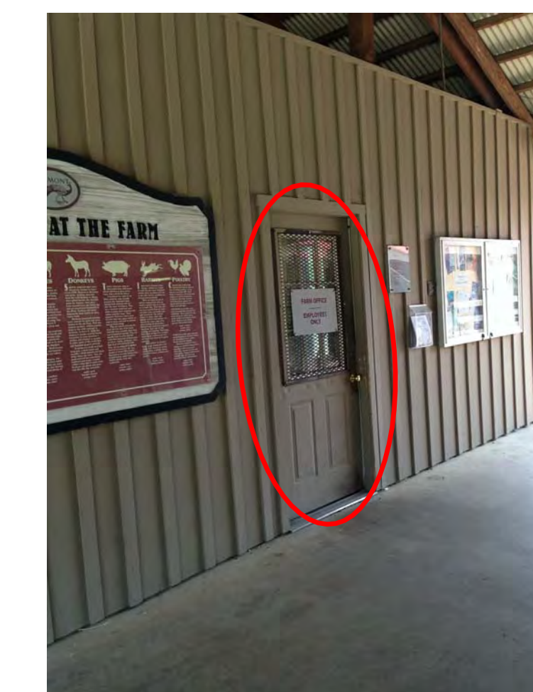
2. REMOVE OFFICE DOOR AND PATCH WALL/SIDING TO MATCH EXISTING
