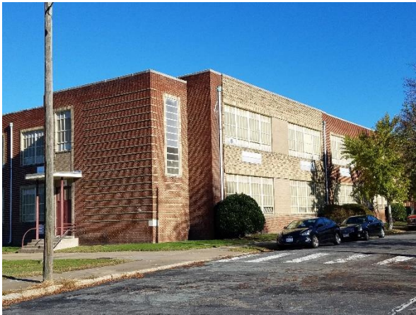
Figure 5. Existing Building, Addition.
